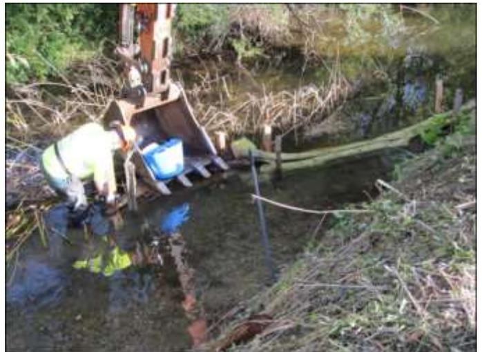
2. Outside edge of berm shaped with locally sourced timber secured by stakes
