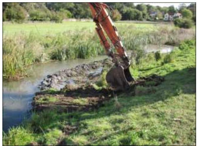
2. Bed material used to define outer boundary of berm
