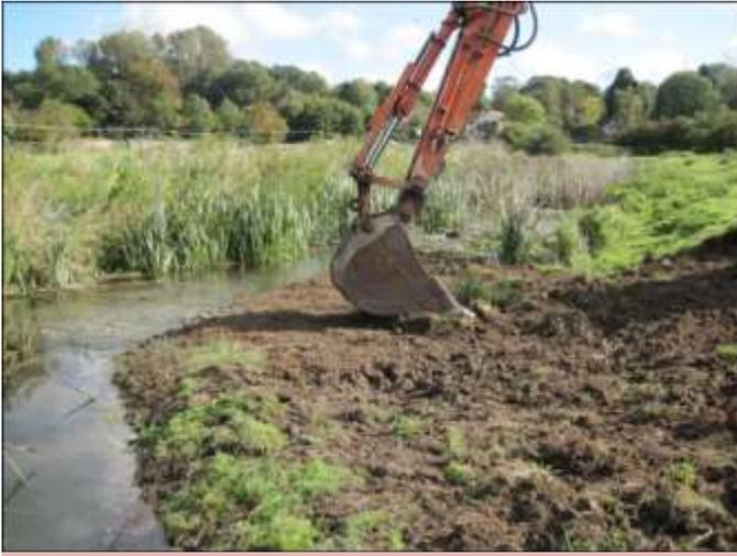
3. Bank re-graded to provide infill material.
