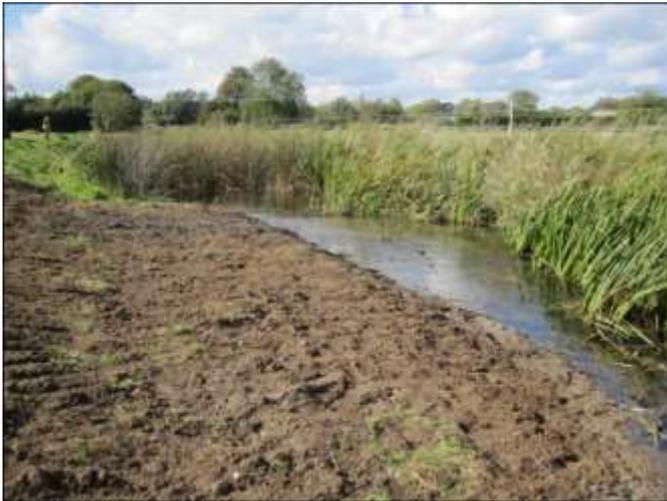
4. Completed berm. Narrows channel at low flows and drowns out at higher flows.
