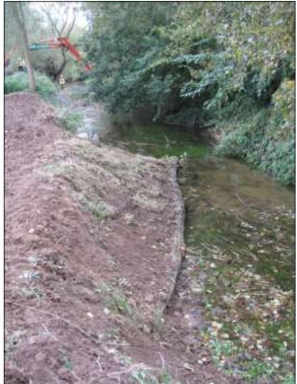
Post-works: channel narrowed and sinuosity increased through installation of berm. Bank re-graded to give gentler slope.
